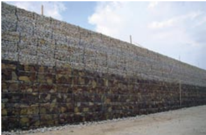
Obr. 5 Múr SO 223 – Terramesh System®
