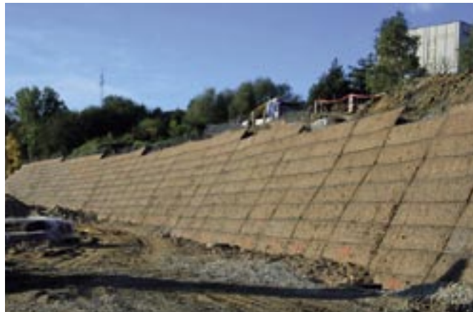
Obr. 7 Múr SO 223 – Terramesh System® SO 269 Green Terramesh s geomrežami ParaGrid®
